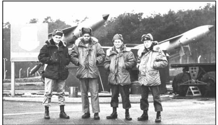
Germany 1-9 crew pictured at the A Flight training pad during construction L to R: Jim Plowden...Tech #2, Bob Simms...Tech #1, Ray Lischka...Crew Chief, Bill Hughes Launch Officer. Photo sent by Jim Plowden
