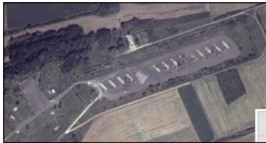
887th the Crown Jewel — All structures gone, area to the lower left was the POL depot area and is now a paint ball arena. Further to the left and just outside the picture was the barracks and Admin area and a bit further on the Grünstadt RC Flying Model Club
