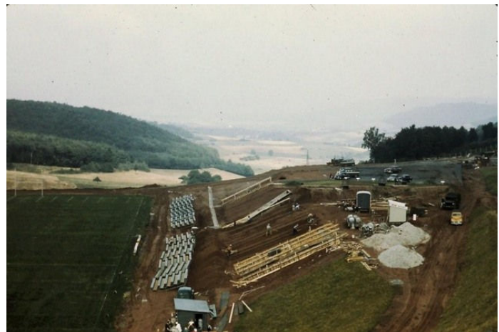
Sembach's Tiger Stadium under construction
